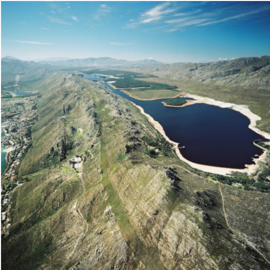
Figure 20: View of Lower Steenbras and the SWTW
