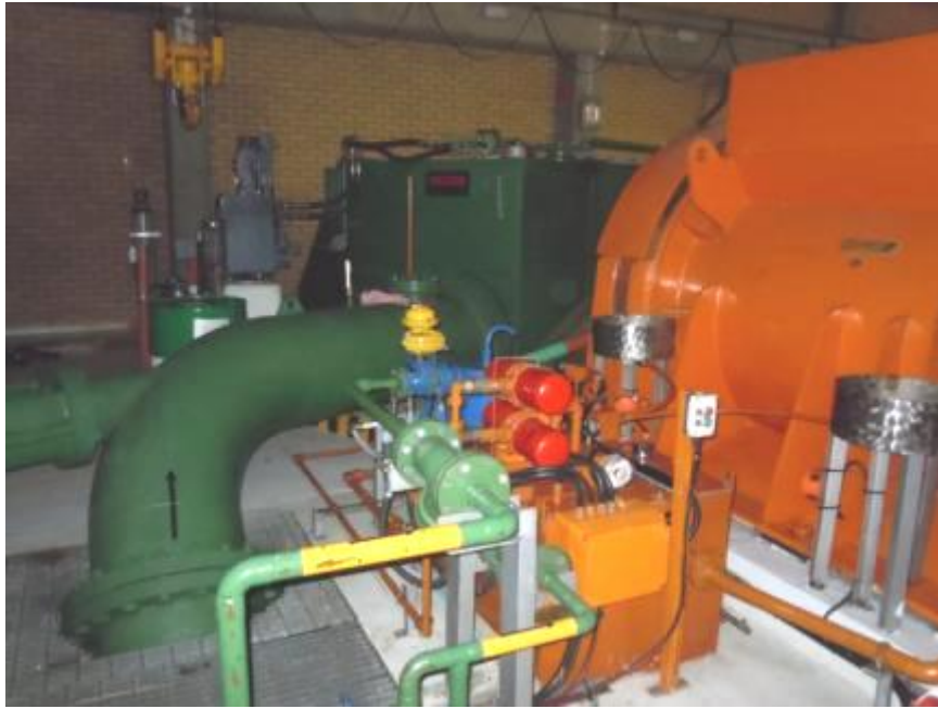
Figure 48: Existing Faure Turgo Turbine
