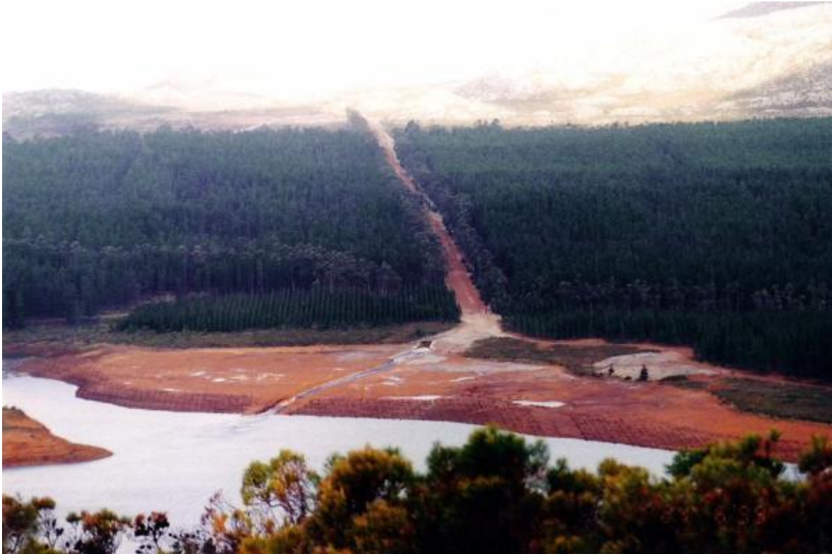
Figure 33: Rockview dam inlet to Upper Steenbras
