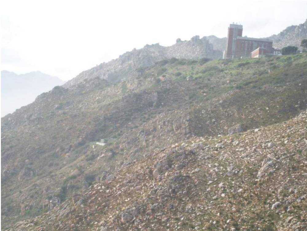
Figure 29: Water Treatment works to upper 760 break pressure tank
