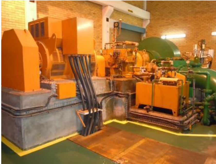
Figure 66: Blackheath Lower Reservoir inlet Turgo Turbine
