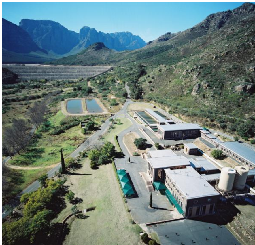
Figure 39: Wemmershoek Water Treatment Works
