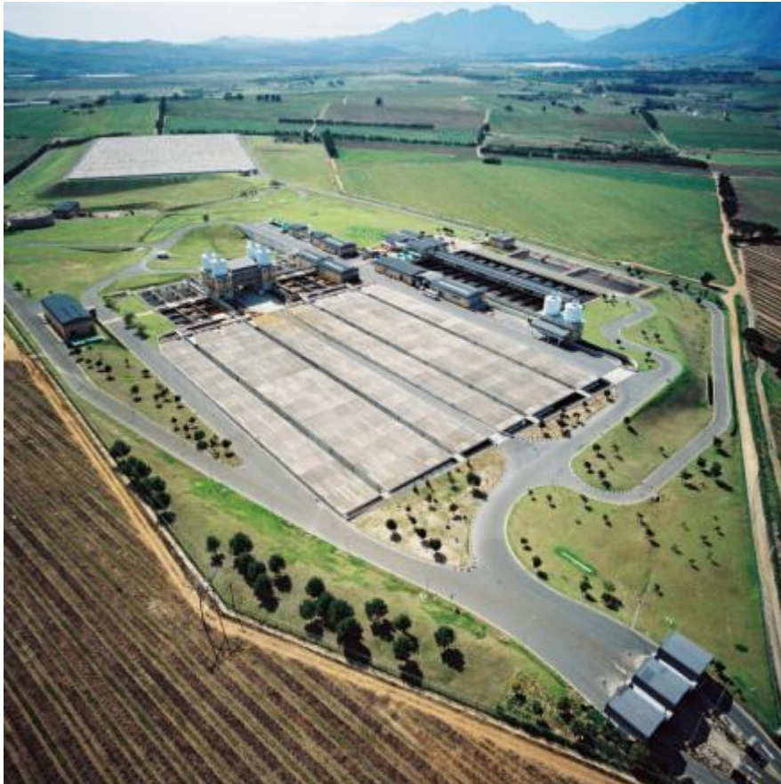
Figure 47: Faure Water Treatment works
