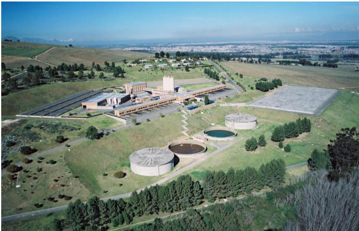
Figure 58: Blackheath Water Treatment Works
