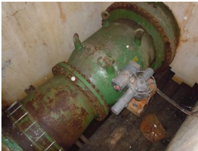
Figure 60: 1100 mm bypass needle valve
