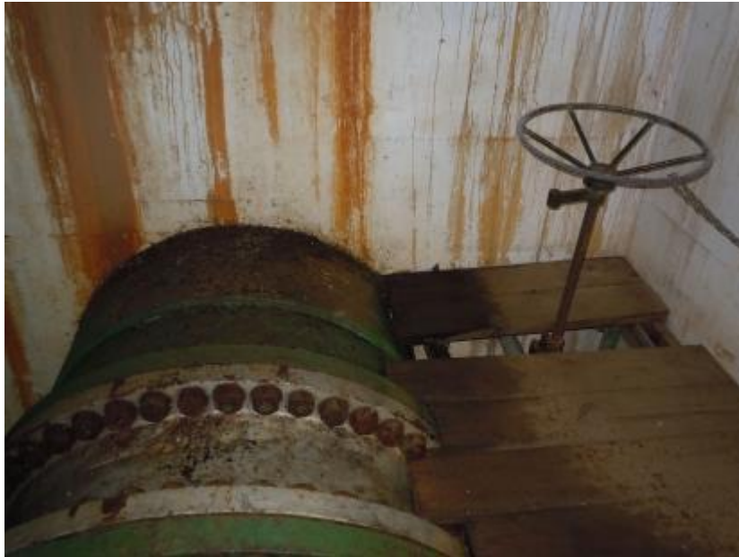
Figure 59: 1500mm needle valve
