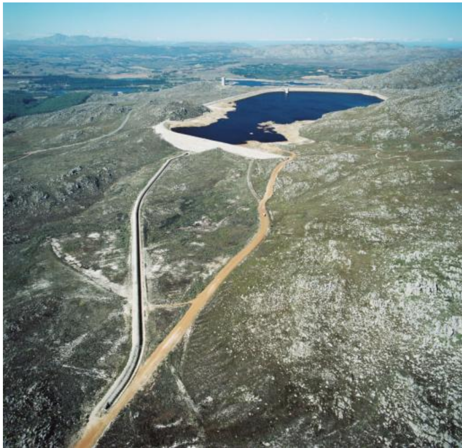
Figure 32: Rockview Dam with canal outlet
