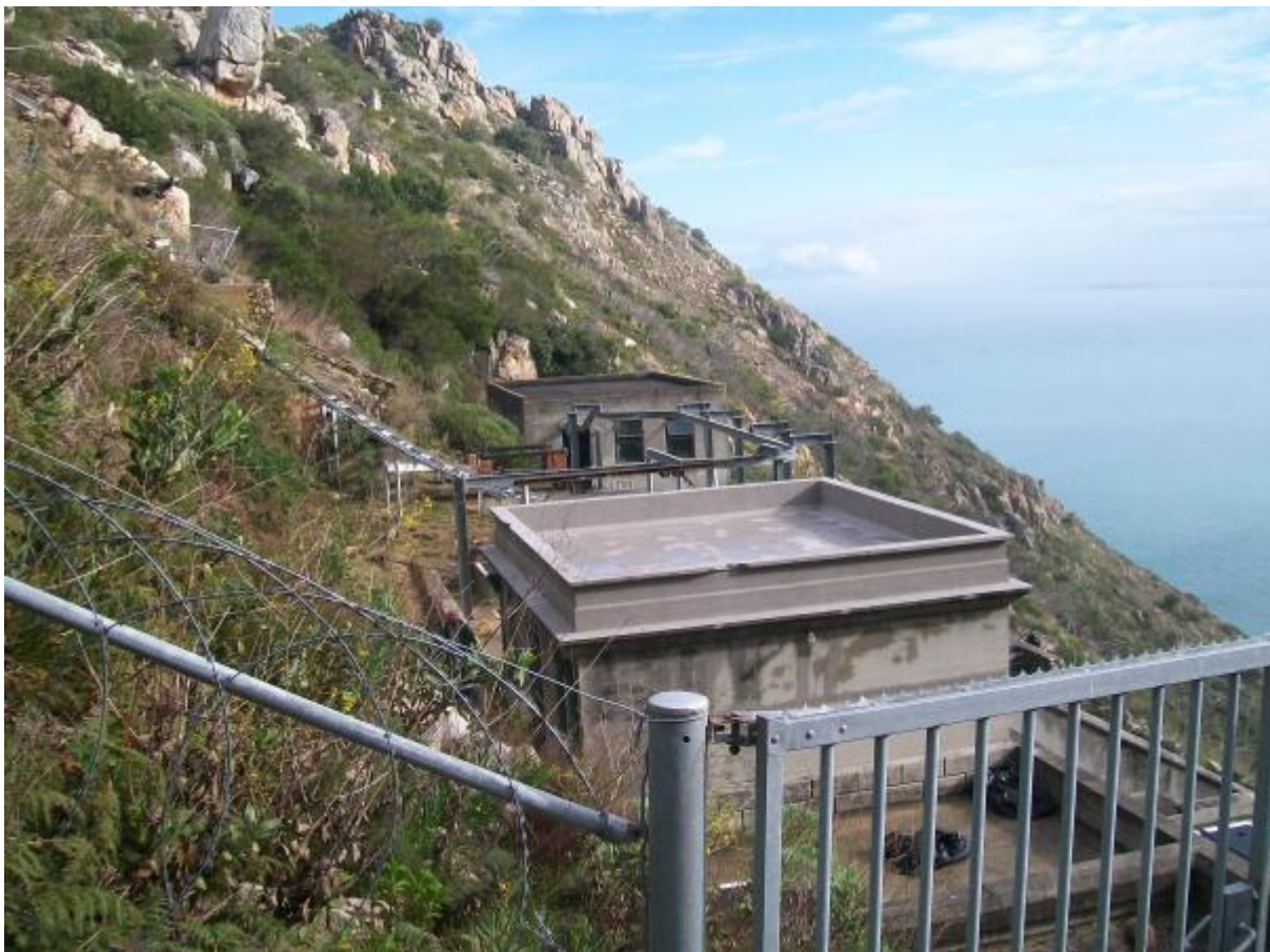
Figure 21: Break Pressure tanks 810 & 840
