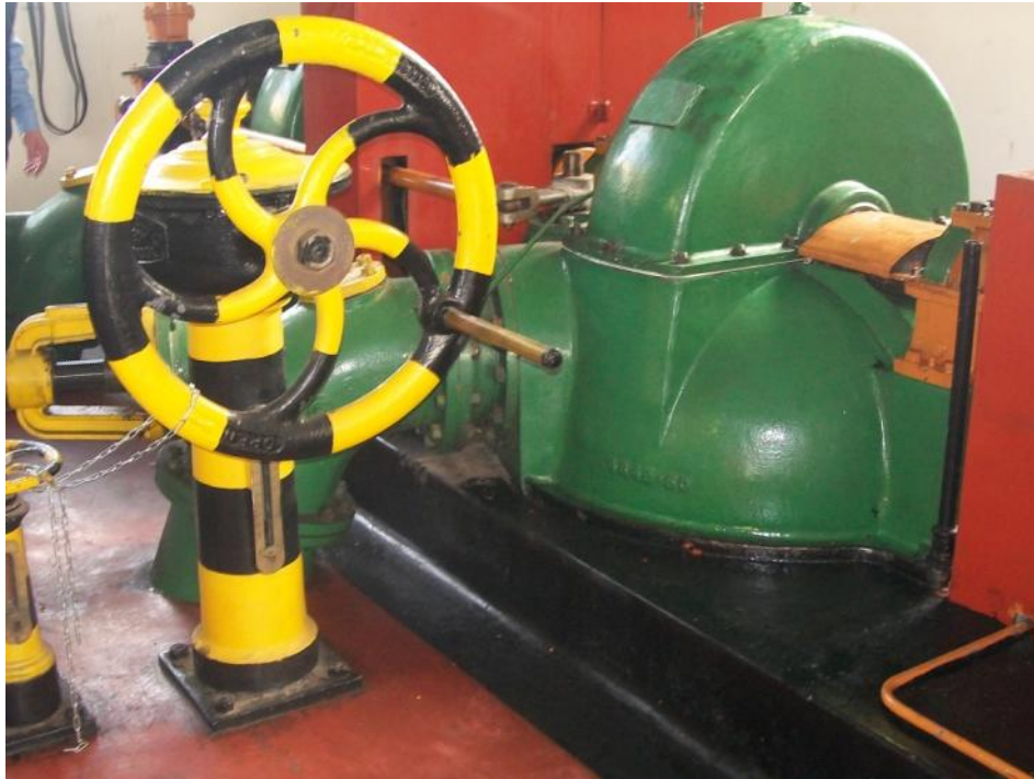
Figure 26: Steenbras Turgo Turbine
