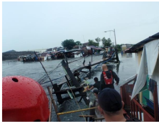
Tabon-Lambingan Bridge destroyed due to raging water along the waterway
