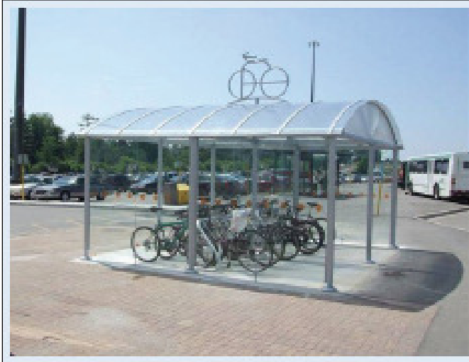
Figure 14. Proper bicycle storage facility at a transit hub in Toronto, Ontario
