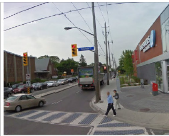
Figure 8. Thermoplastic crosswalk in Toronto, ON (Lawrence at Avenue Rd).
