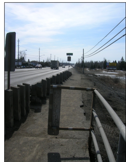
Figure 15. Where the sidewalks ends on the south end of the bridge over the Whitson River near Carol Richard Park.
