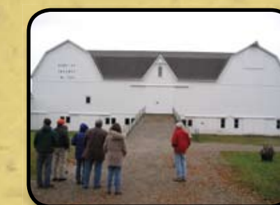
Ellis Barn Springfield Township
