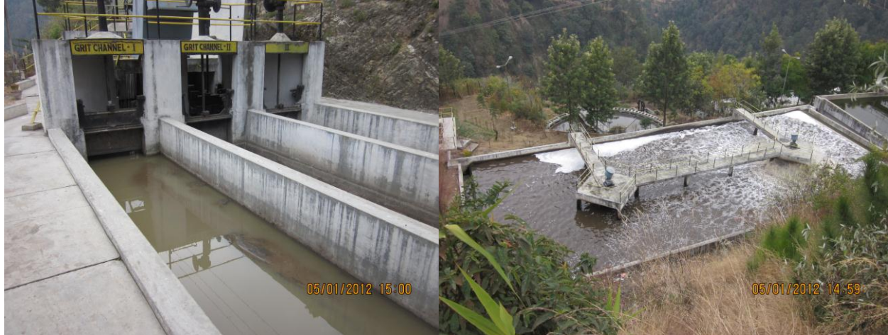
Picture 3: Sewage Treatment Plant at Lalpani, Shimla
