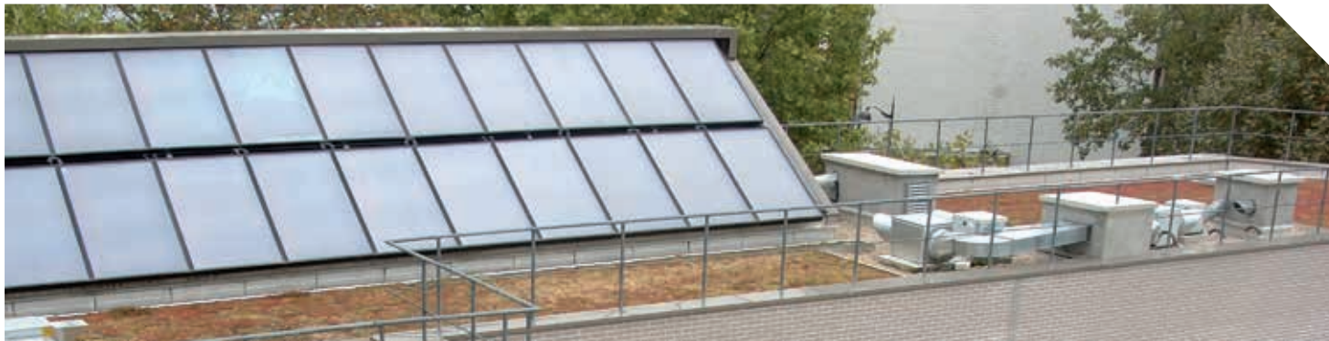
Solar roofing, 19 th
