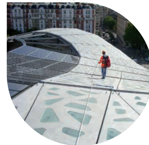
Jean Bouin Stadium, solar panels, 16 th
