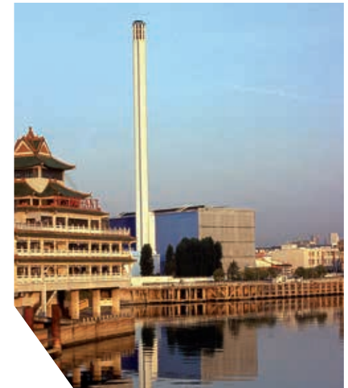
Heat production factory, Ivry-sur-Seine
