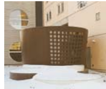
The control room of a wastewater pumping station at Hammarby Gärd.
