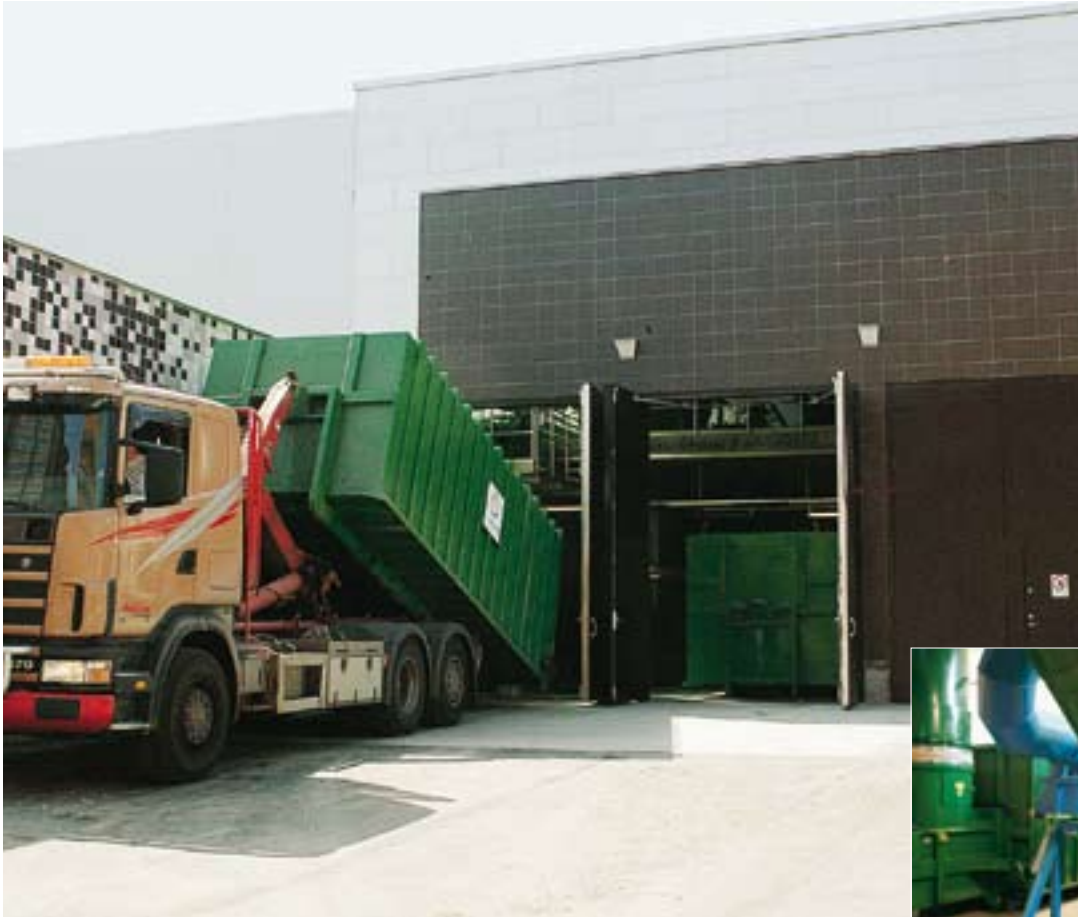
Collection of a waste fraction at the central collection station for the stationary automated waste disposal system at Mårtensdal in Hammarby Sjöstad.
