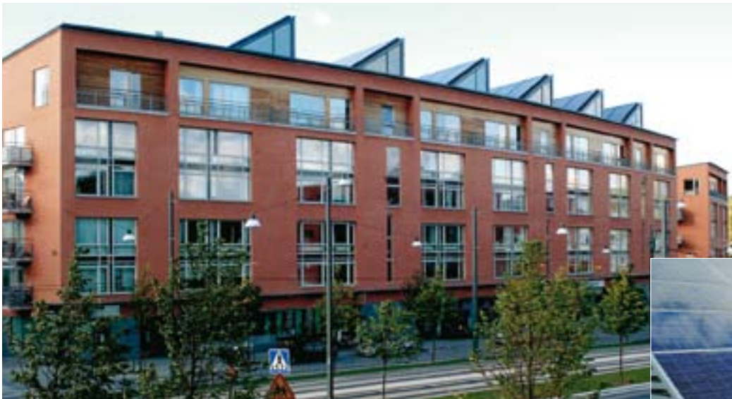
Solar panels. Solar panels that exploit the sun's heat and use it to heat the hot water supply have been installed on many roofs. The solar panels shown in the picture are sufficient to meet half of the building's annual hot water requirement.
