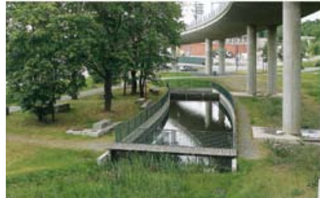
Open storm water basin at Mårtensdal (above).
