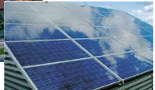
Solar cells. The sun's luminous energy is captured and converted into electrical energy in solar cells. The energy from a 1m 2 solar cell module produces approximately 100 kWh/year, which corresponds to the domestic electricity requirements of 3m 2 residential floor space.
