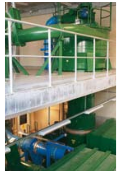
An advanced control system ensures that the waste ends up in the right container in the central collection station.
