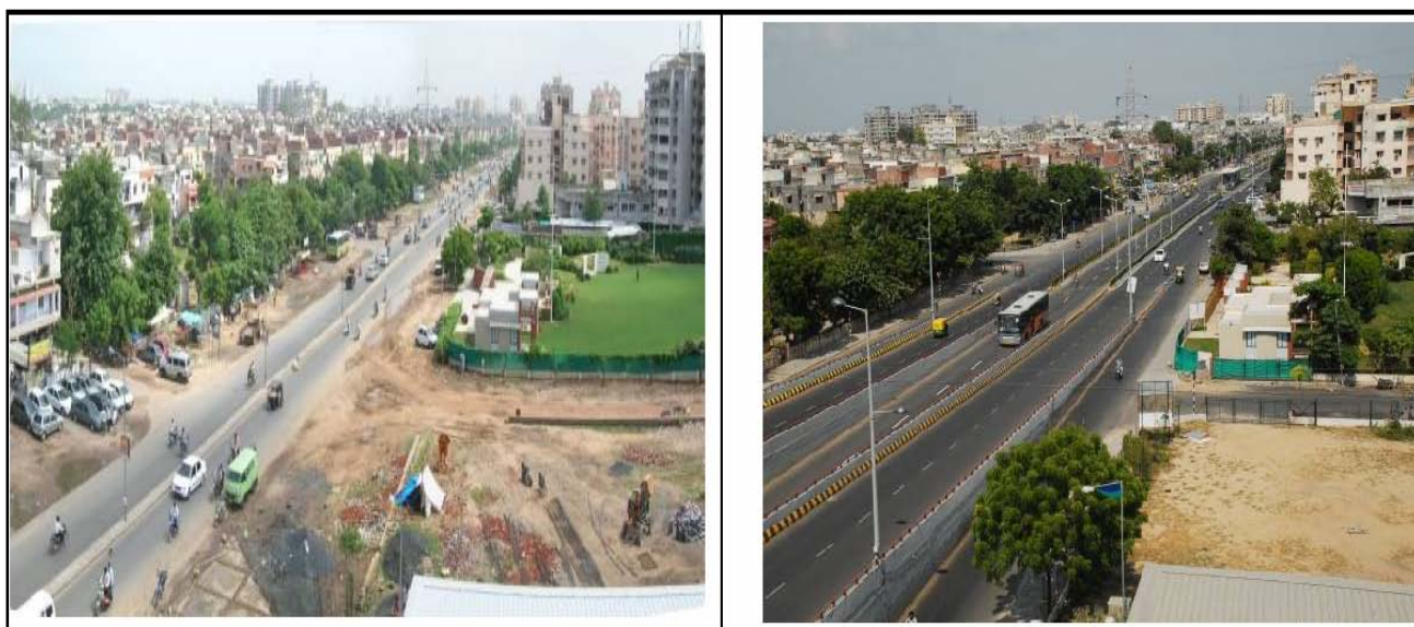
Figure 2.4: Building Split Flyovers (Before and After at AEC)
