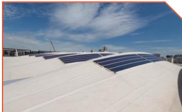
PV cells on gymnasium - 18 th
