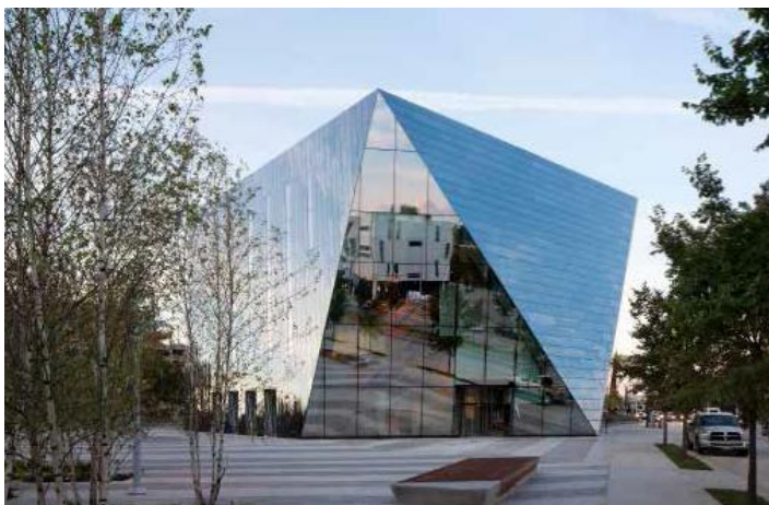
Geothermal systems save energy at the Cleveland Museum of Contemporary Art (Dean Kaufmann, Courtesy of MOCA Cleveland)
