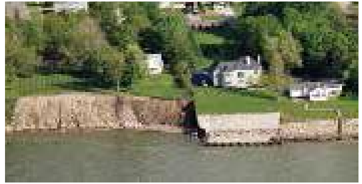
Lake Erie shoreline erosion (Photo: David Beach)
