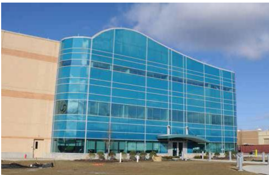
NEORS Southerly Waste Water Treatment Plant - Renewable Energy Facility
