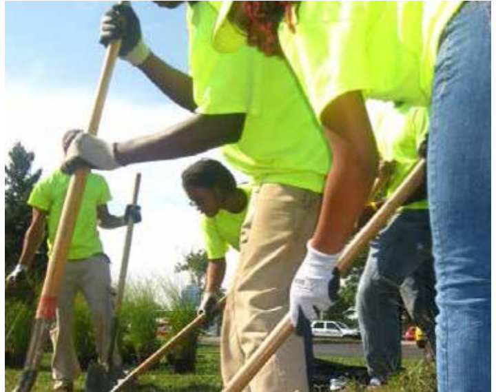
Community Involvement in creating a rain garden
