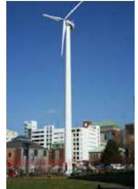
Case Western Reserve University Wind Turbine
