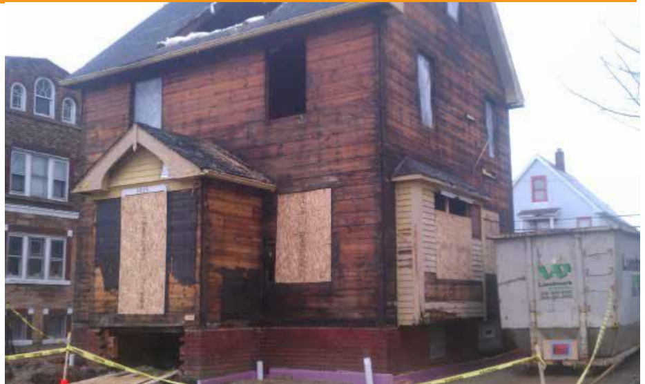
A house before retrofit
