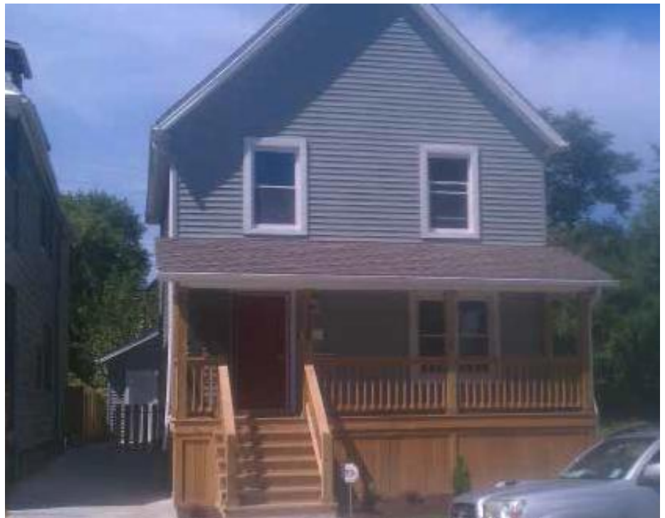
A house after retrofit (Note: The above images are not of the same house)
