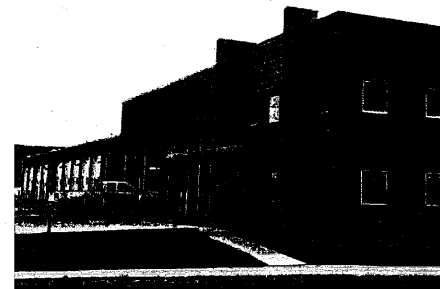
Figure 38. Weather Protection for Pedestrians. (TaigaNova EIP)
