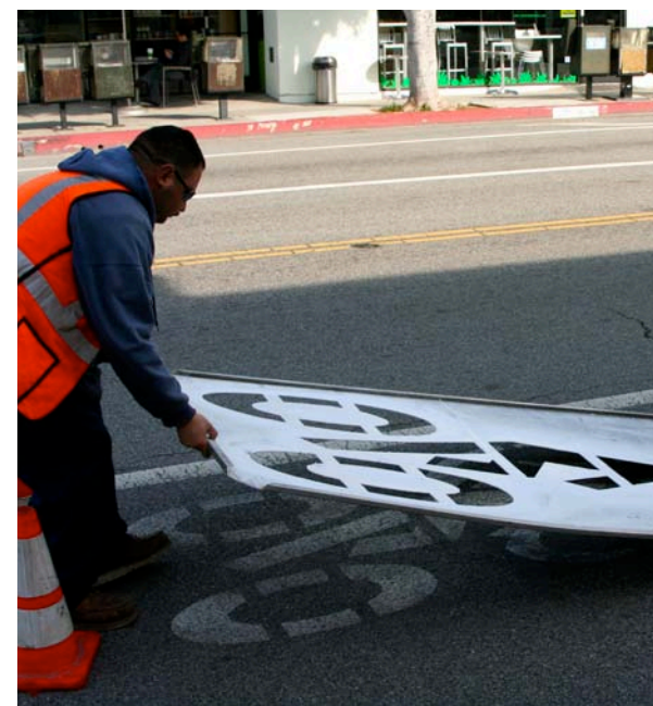
City crews install bicycle lane symbols and directional arrows.
