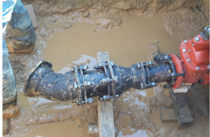
Water main in Baltimore (Source: Flickr user Pam Broviak)
