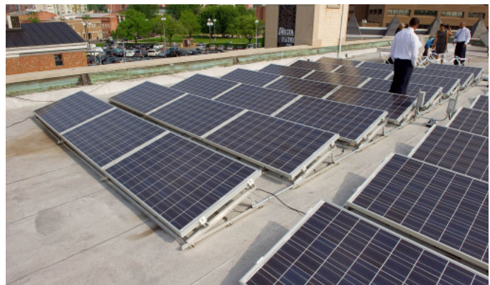
Rooftop photovoltaic installation (Source: U.S. EPA photo by Eric Vance)
