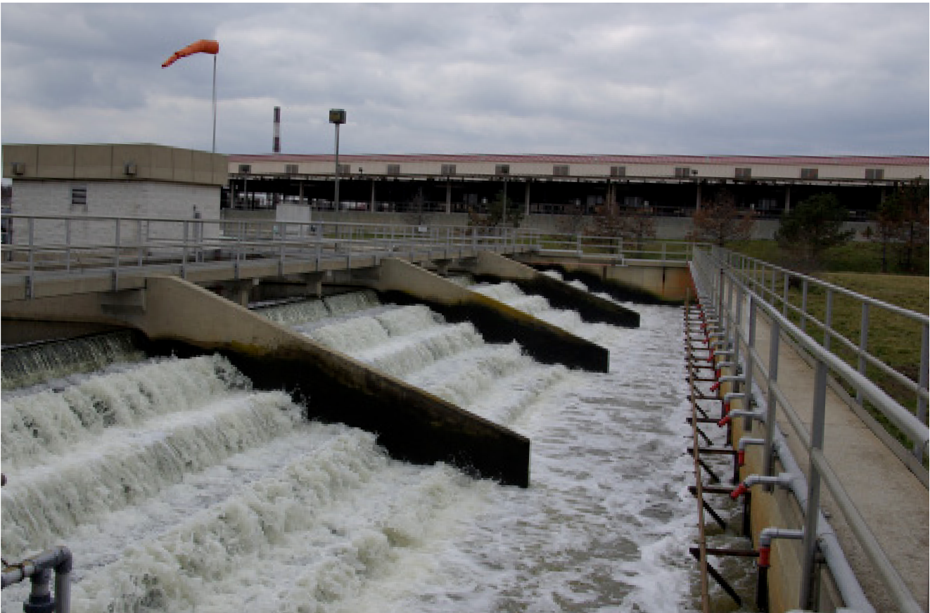
Back River Wastewater Treatment Plant (Source: Flickr User bjorn means bear)
