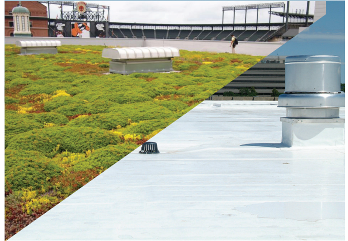
Baltimore Hilton Hotel roof (Source: Baltimore City) (left), White, Reflective, Cool Roof- Tremco HQ (Source: Flickr User Tremco Green HQ)(right)
