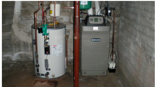
Natural gas boiler (Source: Flickr User Harold Jarche)
