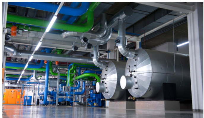
Combined heat and power plant (Source: Flickr User Bilfinger Berger Group)
