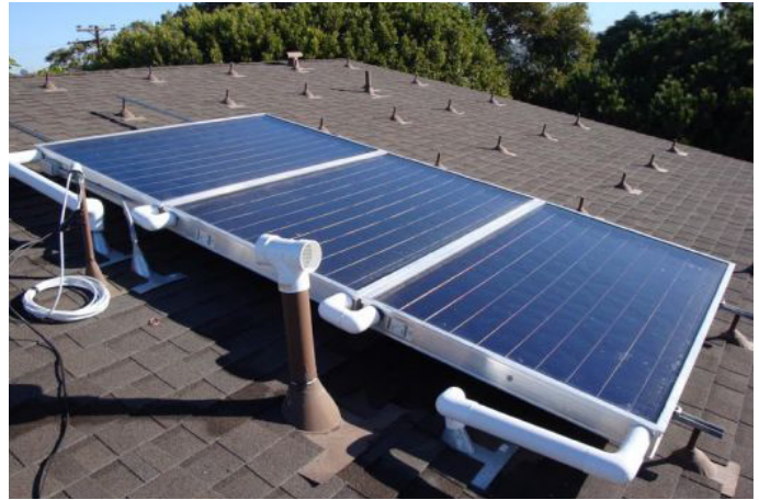
Solar water heater (Source: U.S. Government)
