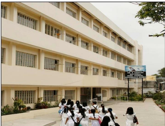
New four-storey High School Building at MOONWALK.
