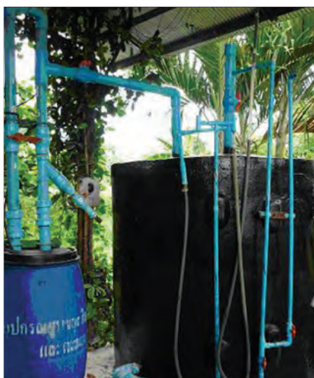
Picture 21. A bio-gas production tank
