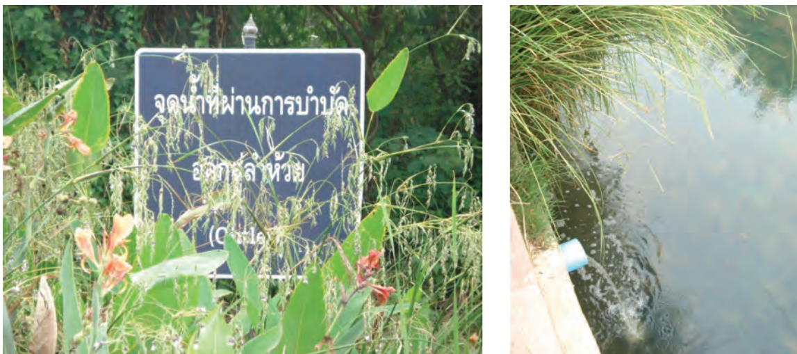
Picture 9: Water treatment outlet
