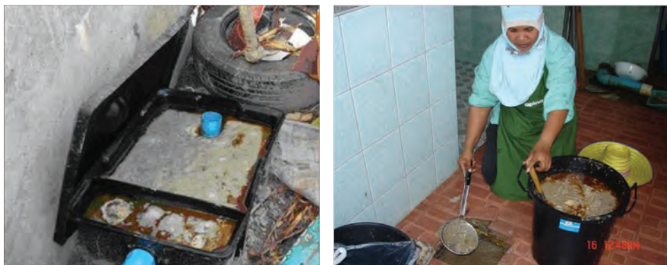
Picture 13. Grease collection simply by hand-scoop
