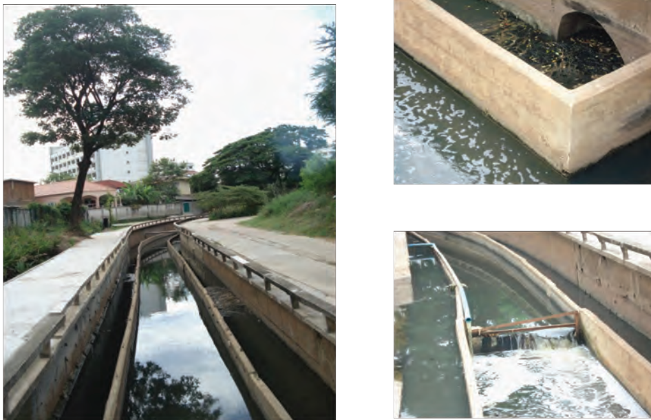
Picture 6: Water diversion way in creek for divided wastewater and treated water
