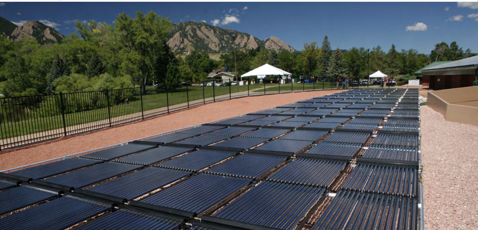
Solar thermal system at South Boulder Recreation Center.
