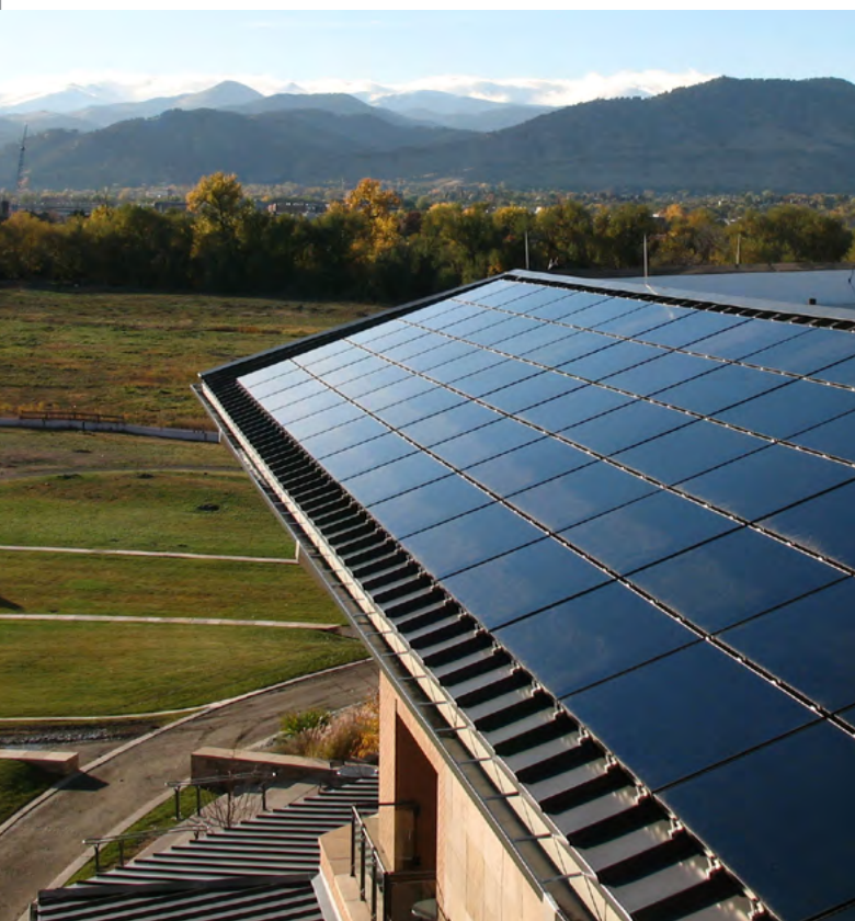
New solar PV array at Boulder Community Hospital, part of Boulder's 11.3 MW of site-based solar generation
