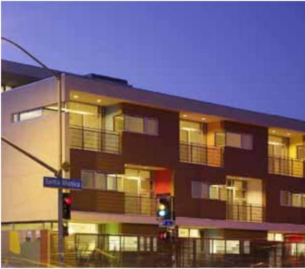
Affordable and workforce housing is highly desirable.
