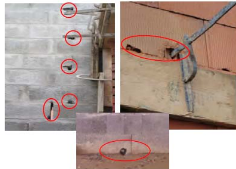
Walls are damaged by construction clamp
