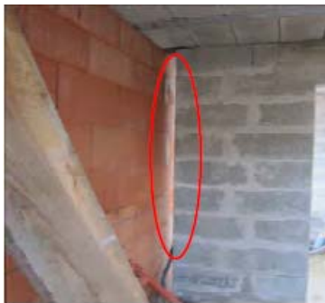
Walls inside the house is separated from the exterior wall
