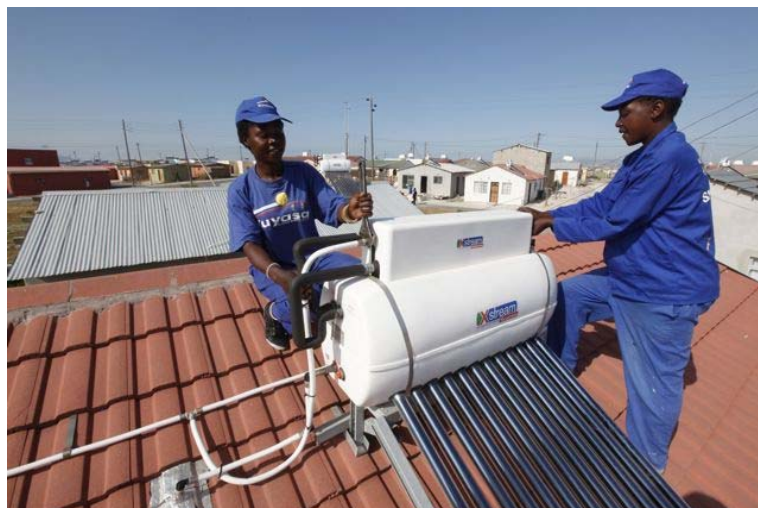
Figure 2 Locally manufactured SWH in Kuyasa
