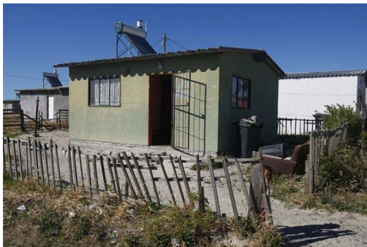
Figure 1: Typical RDP house in Kuyasa
