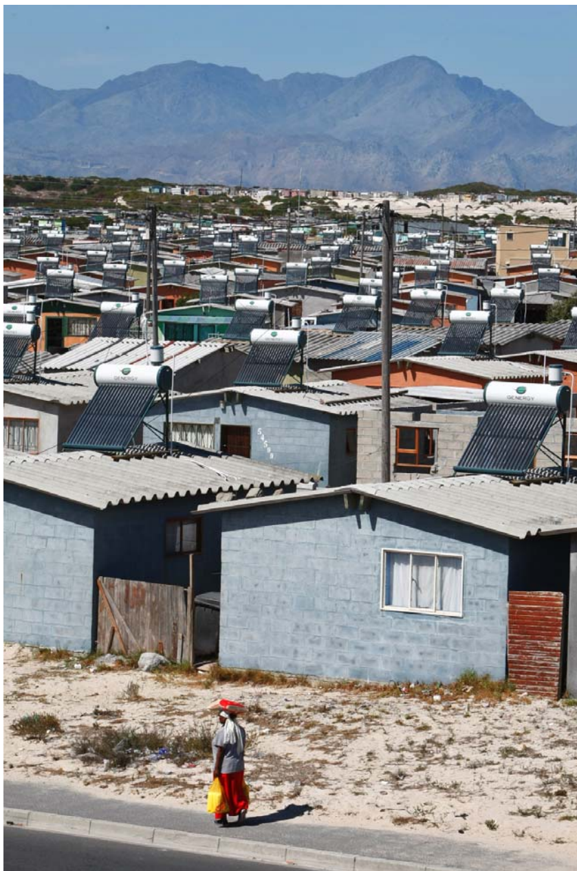
Figure 18: The community of Kuyasa after project completion
