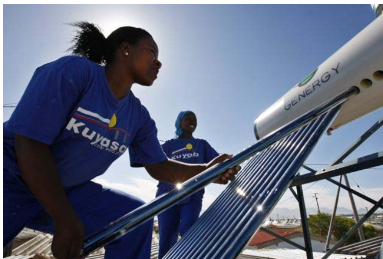
Figure 10: SWH installation
