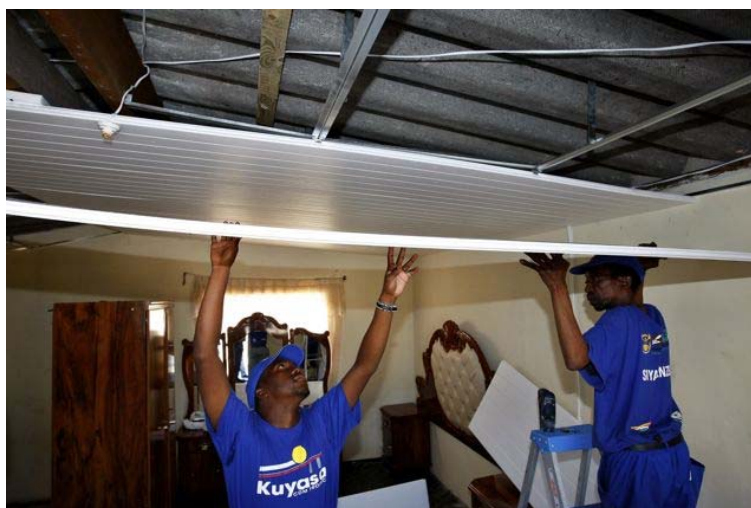
Figure 9: Insulated ceiling installation
