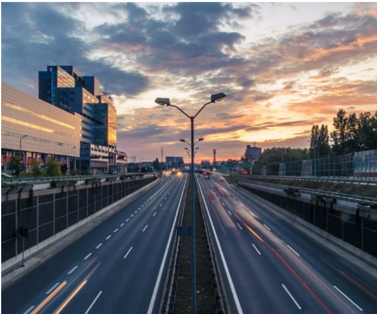
City of Katowice, Poland.
